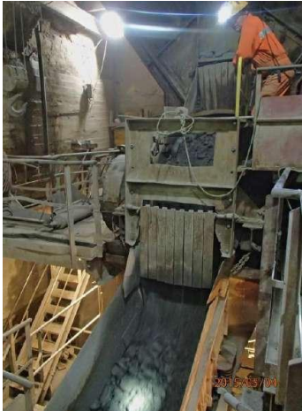
Underground crushing chamber
