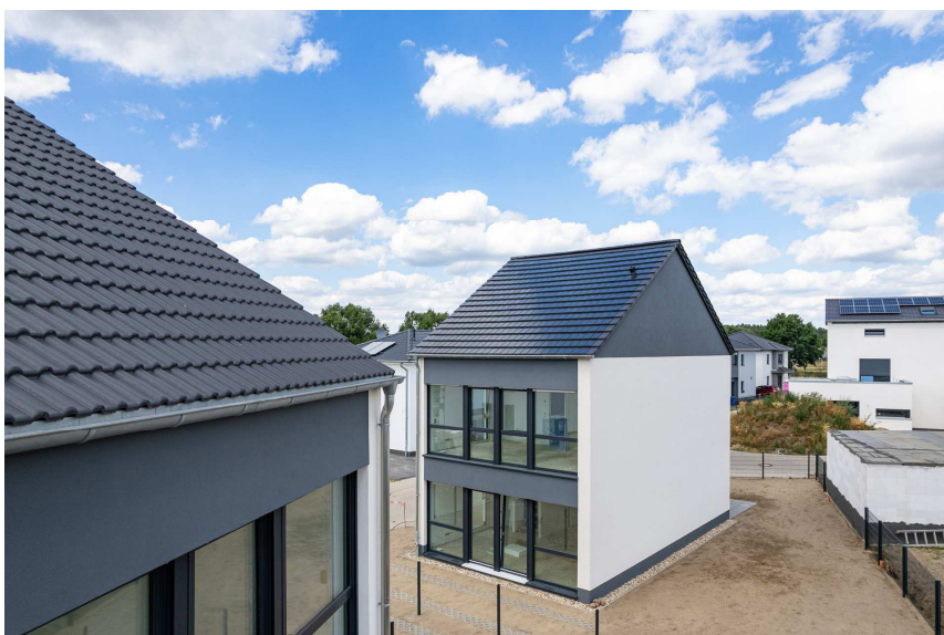
Figure 2: Terrabau: Green home construction
